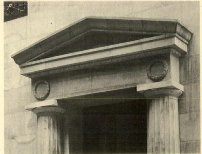
Bank Building of Lee, Higginson & Company New York City Cross & Cross
