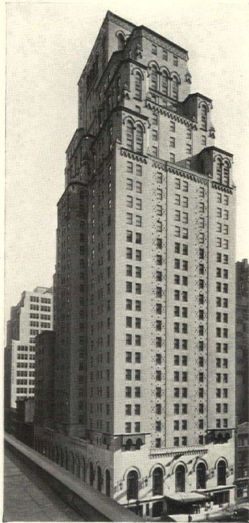
THE HOTEL GOVERNOR CLINTON, New York City Murgatroyd & Ogden, Architects
